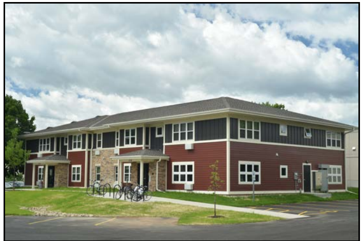
Thierer Road – 28 efficiency apartments
